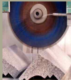
Diamond Saw Cutting
